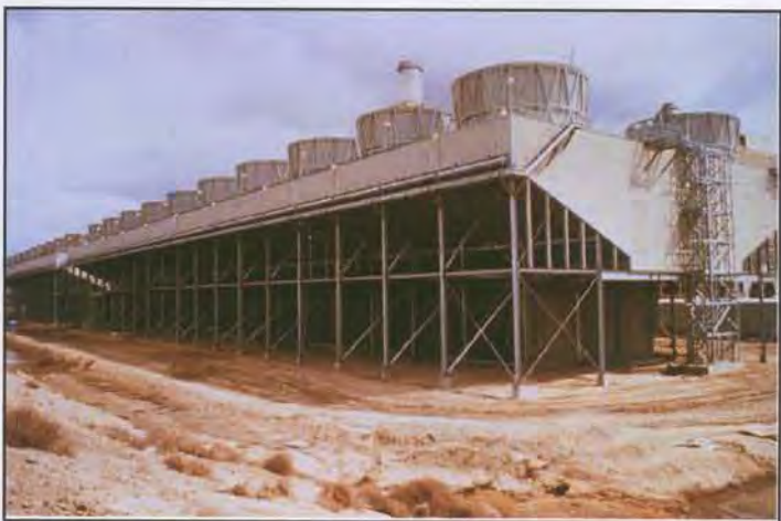
Figure 7. Water conservation tower on a power plant
