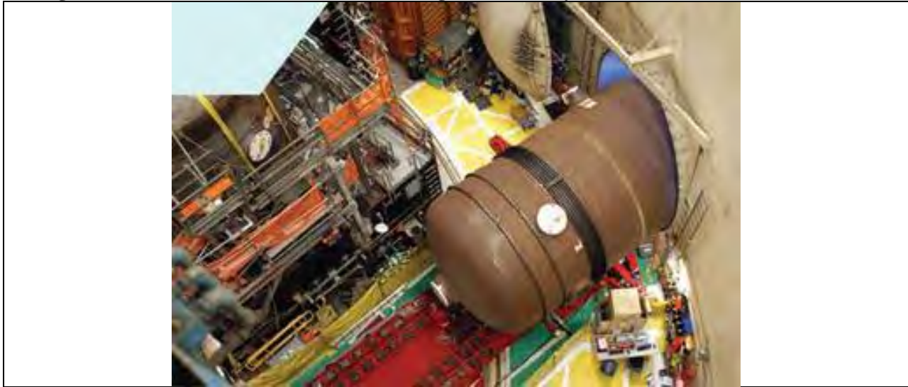
Figure 12. New Steam Generator Entering Diablo Canyon Unit 1 Containment Dome 55
