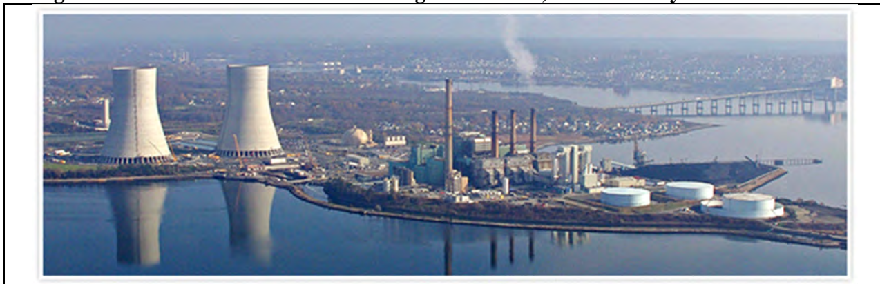
Figure 13. Retrofit Natural Draft Cooling Towers at 1,500 MW Brayton Point Station 59
