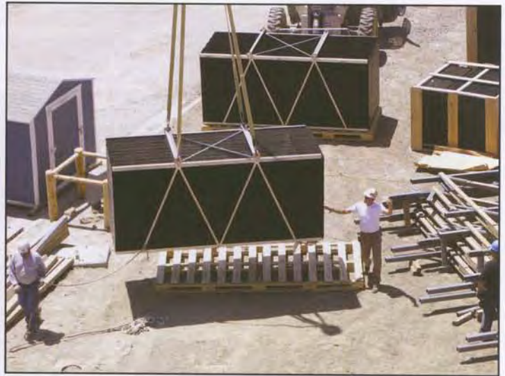
Figure 13. Hoisting of factory assembled condensing modules [photo by Dennis Parker]
