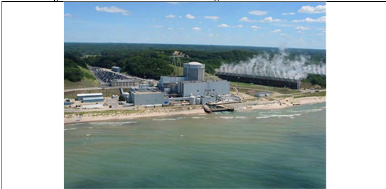
Figure 2. Mechanical Draft Inline Cooling Towers at Palisades Nuclear 14
