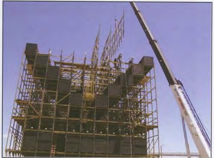
Figure 14. Tower under construction, showing position of modules [photo by Dennis Parker]
