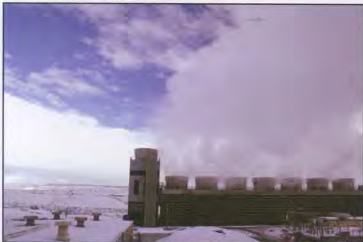
Figure 17. Cold operation of the demonstration cell [Date 2/09/09 Temperature 35°F Relative Humidity 50%, photo by Jared Hickman]
